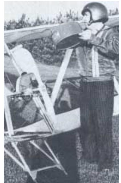
**Mix of 100-octane gasoline** and synthetic oil fuels the little engine. Moody reports no plug fouling with this mixture. Special 28-inch-diameter prop has very low pitch.
